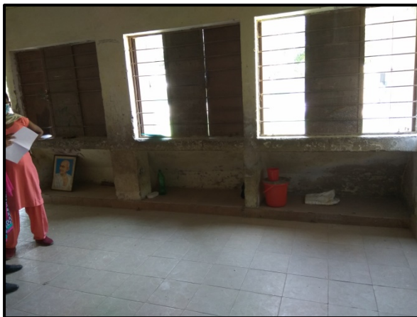
Open slabs at Nayabans AWC No- 5
