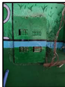
Switchboards at Mangroli AWC No.
