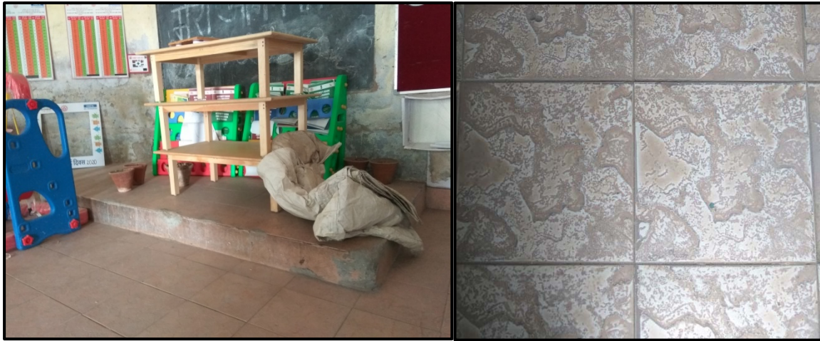
Tiled flooring at Nayabans AWC No- 5
